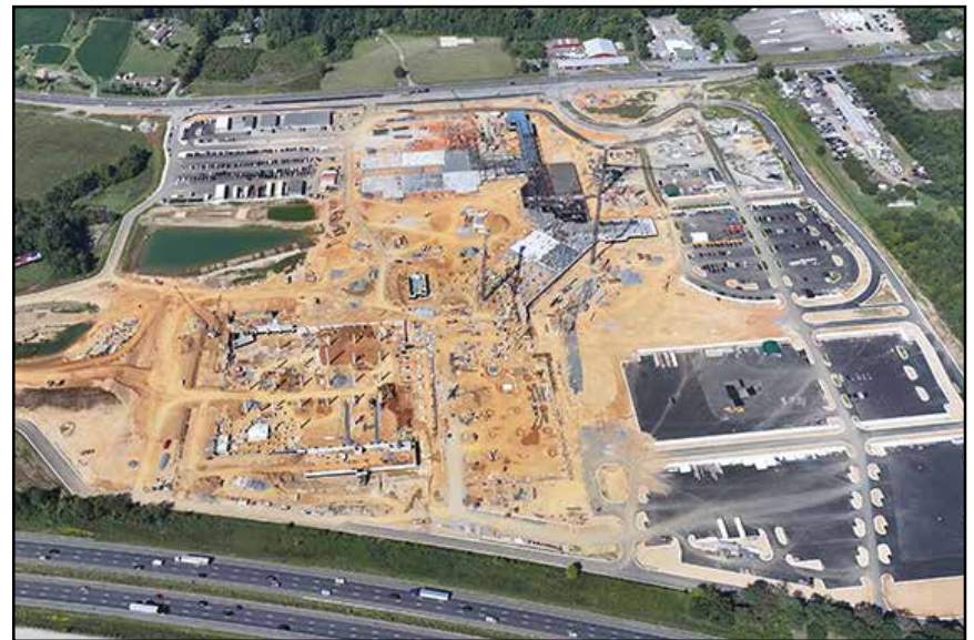
Aerial photo of Kalahari site at Thornburg next to I-95.
