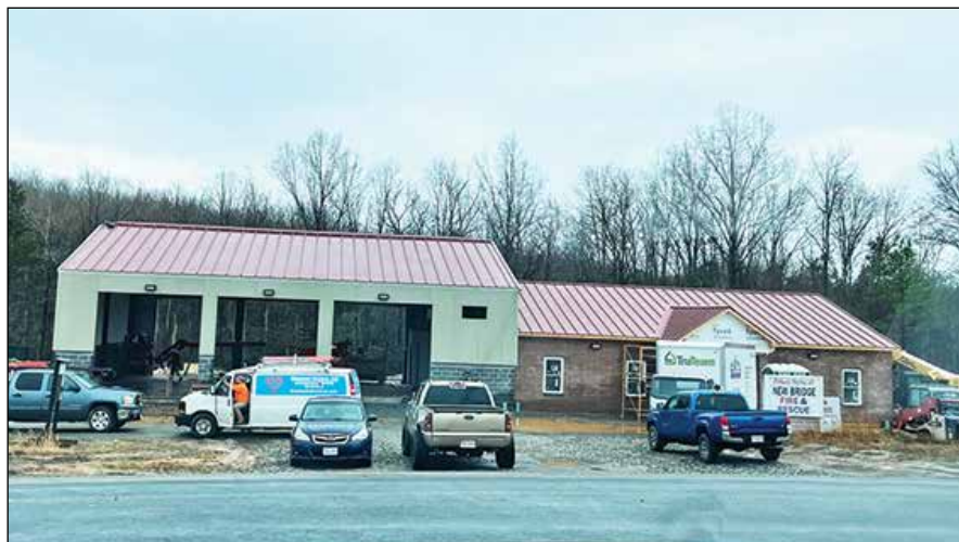
New Bridge Station 8 in February.
